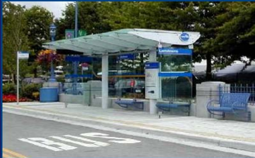
Number Three Rd Transitway Vancouver 98B
